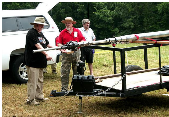
Field Day 2012 WA4AHR, W4ORD, and WD4CEE setting up Dewey's home built crank-up tower Picture courtesy of KK4BPH
