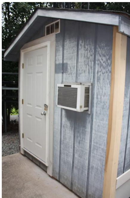
The shed showing new door and some of the repairs.
