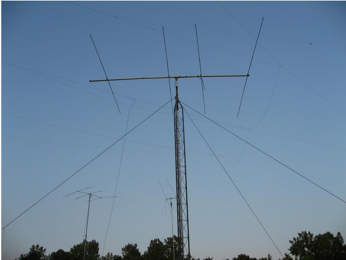
Towers set up just before sunset Friday: Front – W4BOH's tower for the 10m yagi; Rear left: W3AHL's 55' crank-up tower for 20m; Center bottom: KV7D's crank-up tower with the 15m cubical quad; Not yet up, W4BOH's trailer based tower for a 15m beam. You might also be able to see KV7D's wire yagi above it all.
