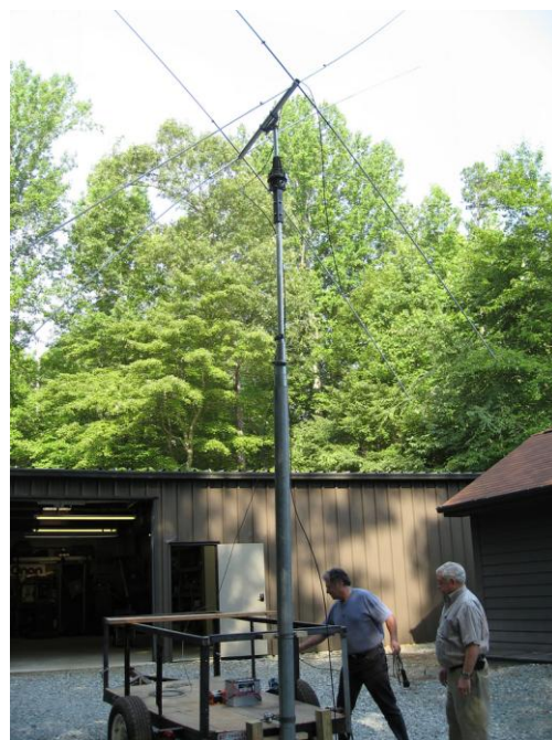
Adriano, KV7D, and Dewey, WA4AHR, putting the finishing touches on their DIY crank-up tower.
