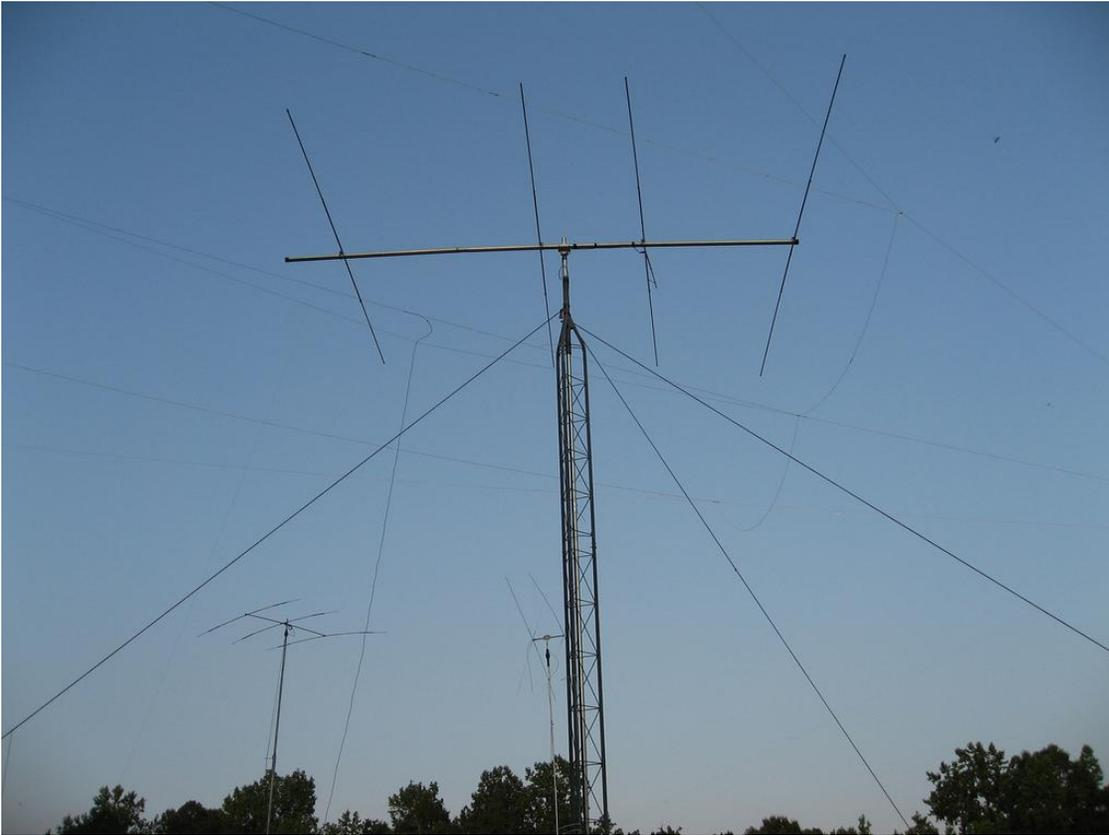
Towers set up just before sunset Friday: Front – W4BOH's tower for the 10m yagi; Rear left: W3AHL's 55' crank-up tower for 20m; Center bottom: KV7D's crank-up tower with the 15m cubical quad; Not yet up, W4BOH's trailer based tower for a 15m beam.
